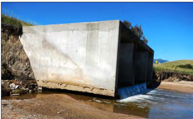
Vehicles on State Highway 128, southeast of Boulder, regularly travel over this concrete box culvert, which faces scour concerns. At the culvert outlet, water has eroded three feet from the bank of Coal Creek.
