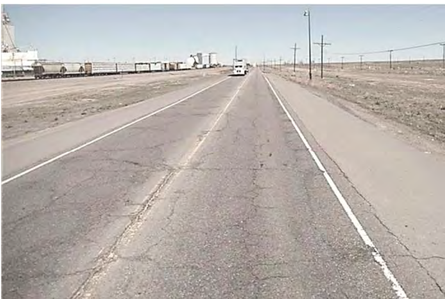
This stretch of pavement, on State Highway 2C at the northwest boundary of Rocky Mountain Arsenal National Wildlife Refuge, has a Drivability Life of zero years. Extensive surface cracking is one factor placing the pavement in the Low Drivability Life category.
