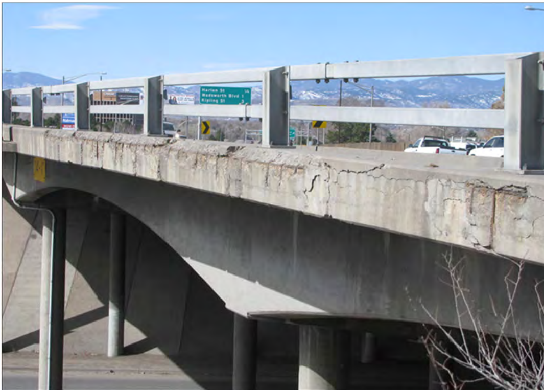
A deteriorating overhang on a bridge on Interstate 70, near Lakeside Amusement Park in Denver. CDOT maintains this bridge that was built in 1966, ensuring that concrete does not fall on vehicles traveling underneath.
